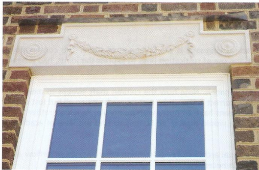
This photo taken during construction shows a hand-carved limestone window header for an English Georgian, circa 1720–1760. Note that the lead-coated copper flashing remains yet to be trimmed and finished.
